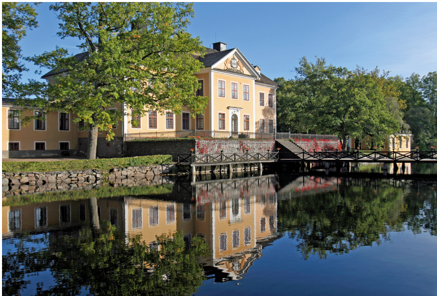
Leufsta Bruk manor house as seen from the north.
